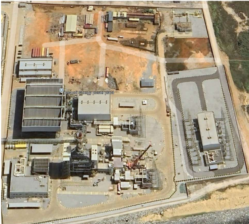
200 MW Amandi Energy Power Plant, Ghana
